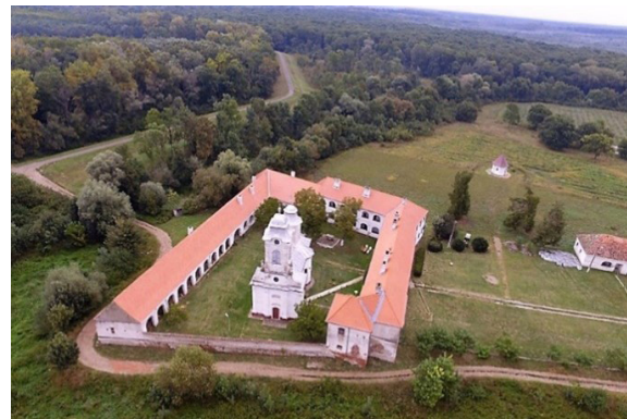
Fig. 1. Aerial view of the Bezdin Monastery
