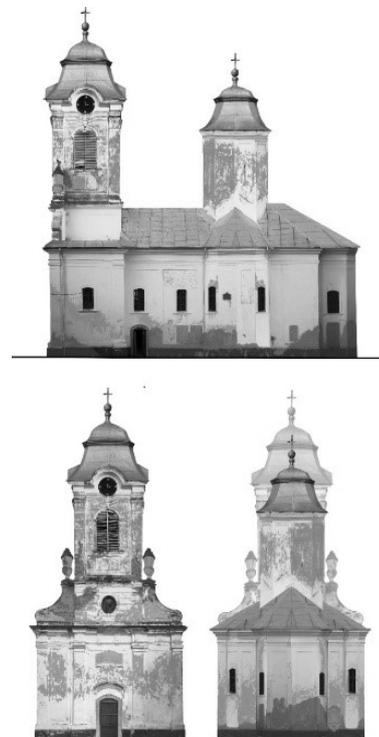
Fig. 3. 3D laser scanning of Bezdin church – façades
