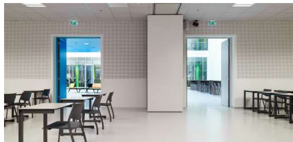
Fig. 19. Mobile wall finished with laminated composite material [16]
